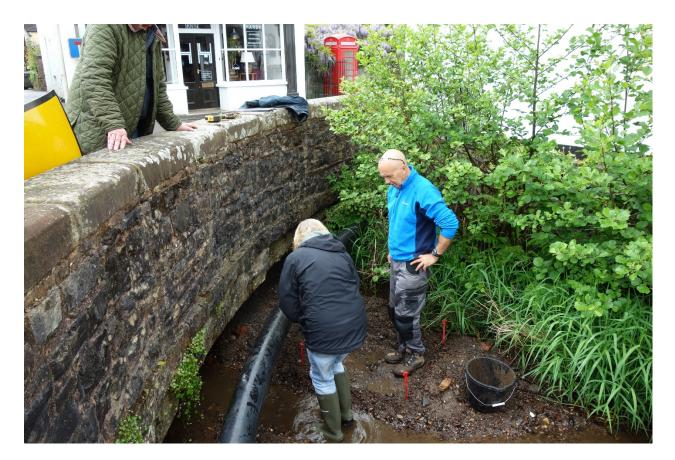
Figure 2 – Marking out the trench.
